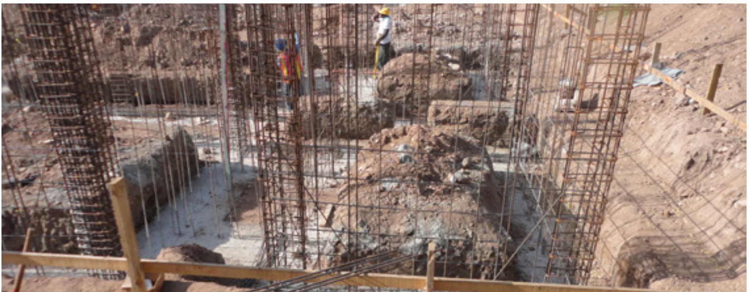
Construction in Progress
