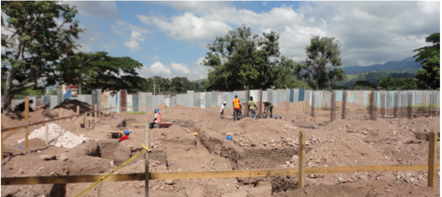
Construction in Progress
